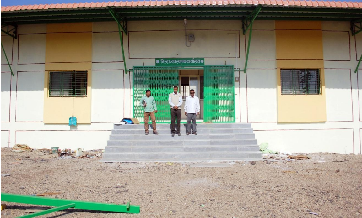
Seed Processing Plant, MSSCL, Hingoli
