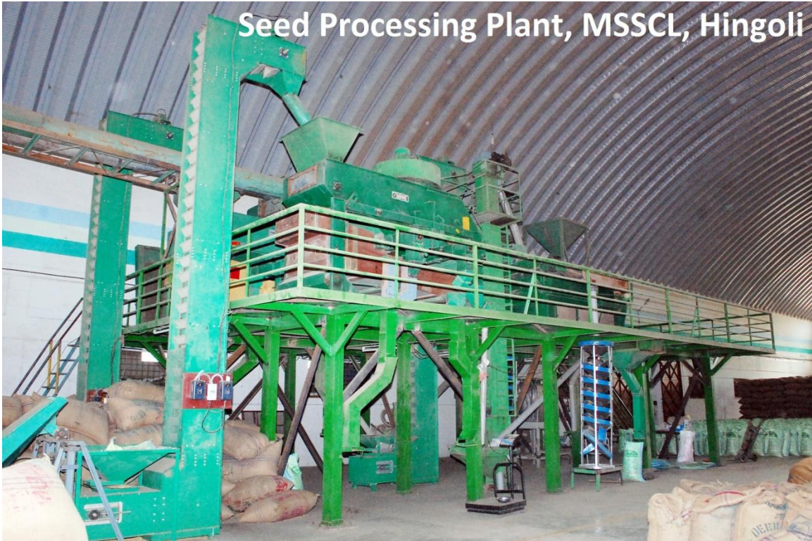
Seed Processing Plant, MSSCL, Hingoli
